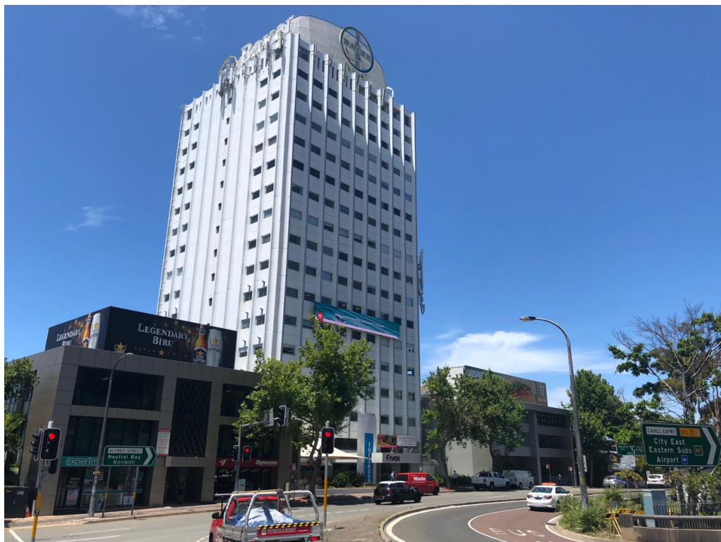
Figure 5 – Built form along Alfred Street Source: Grimshaw
